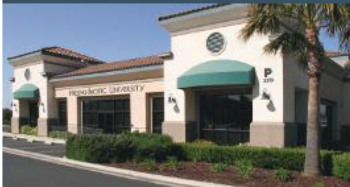
Fresno Pacific University's new 4,800-square-foot Merced Center.
