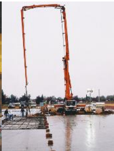
Glendon Becker, auxiliaries director and Pacific Bookshop manager, looks over plans for Alumni Hall inside the reconstructed building. Right, machinery at the Haak Tennis Complex included a rig that can pour concrete anywhere on the site from one location.
